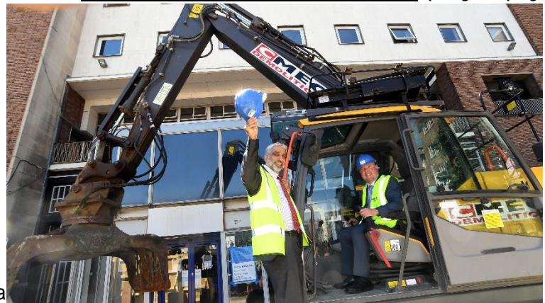
The demolition will re-establish the link between Broadgate and Hertford Street
